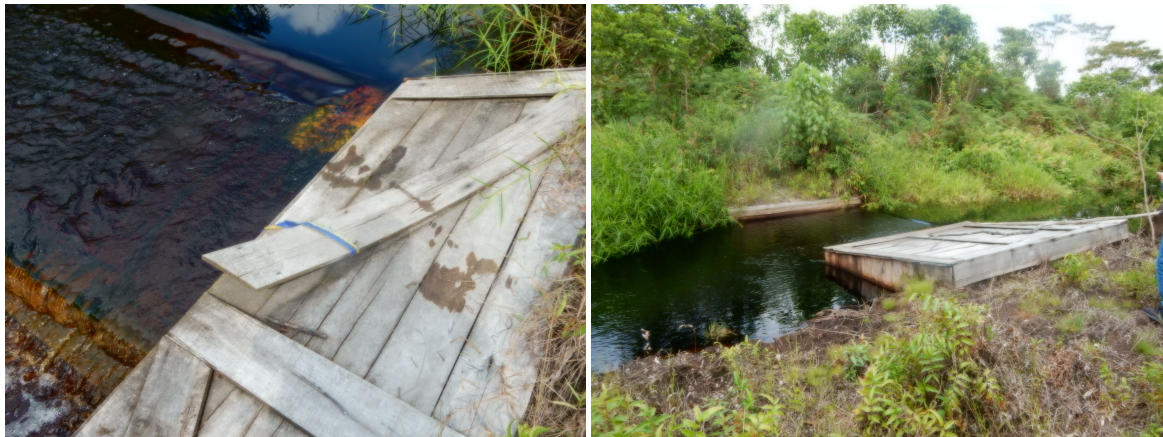
Figure 6. WWF Dam and Deteriorating Wood
